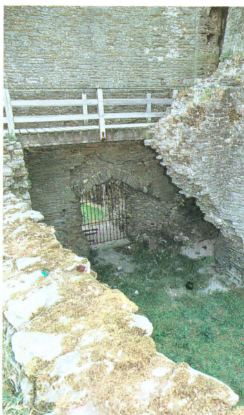
The spillway at the southern end of the north dam was designed to take floodwater from the castle lakes.
