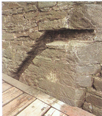
One of the unusual drawbridge sockets to be seen in the side walls of the main outer gatehouse.
